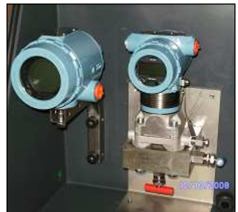
ENCLOSURE S3-1 with window Example for Emerson 3051CD and 3144P
